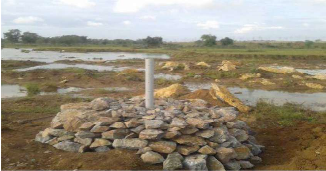
Figure 1- Recharge Well No 1
