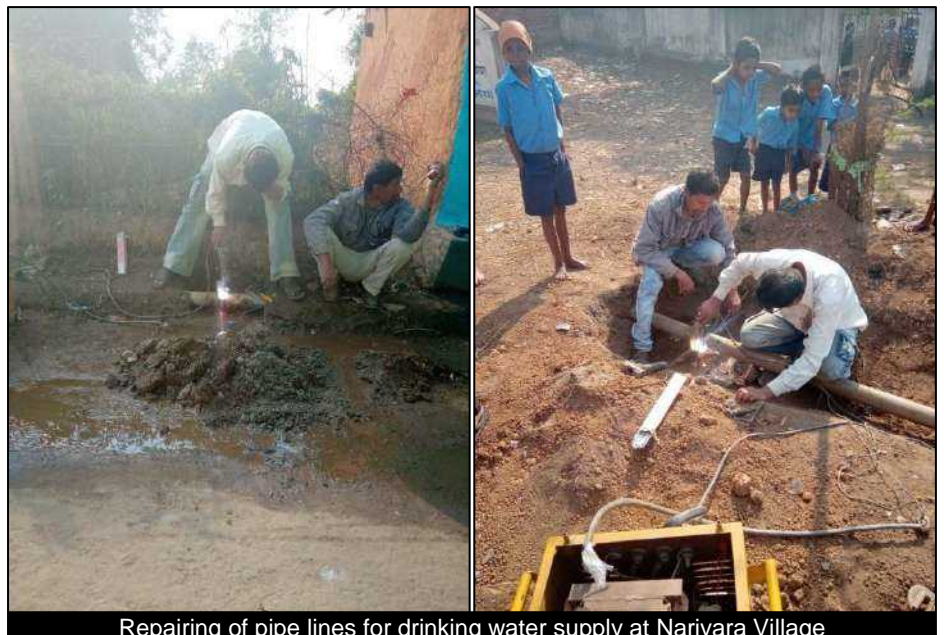
Repairing of pipe lines for drinking water supply at Nariyara Village
