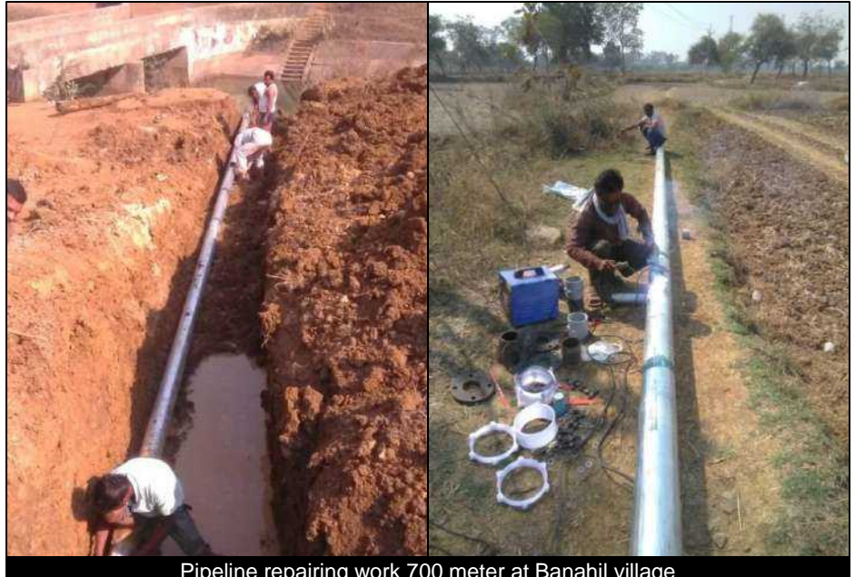
Pipeline repairing work 700 meter at Banahil village
