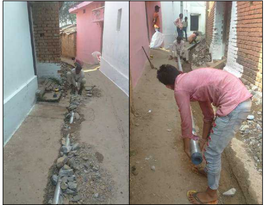
Pipe Line Extension work 638 meter Gram Panchayat Banahil
