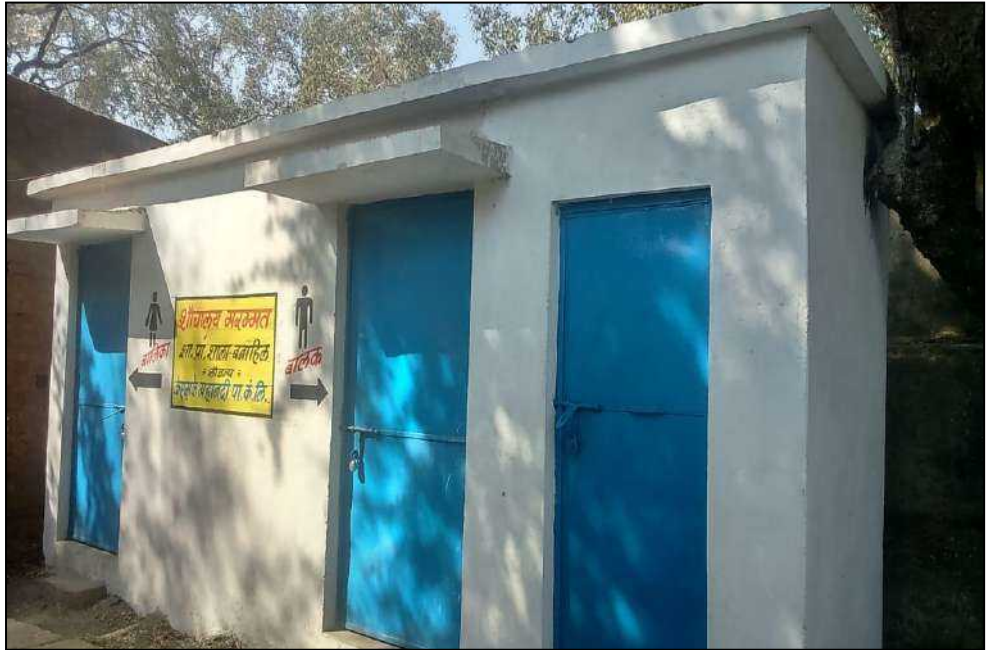
Urinal-Toilets new Construction and Repairing work at Govt. primary School Banahil
