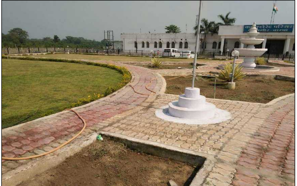
Submersible Pump, Grass Cutter Repairing and Beautification at Collectorate Garden Janjgir
