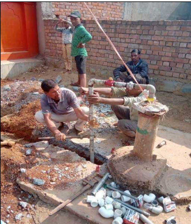
Connecting of the Submersible pump to pipe line work, ward no 13, and 14 at Nariyara village
