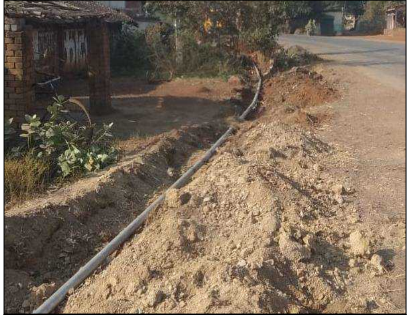
Pipe Line Extension work 1101 meter Gram Panchayat Nariyara
