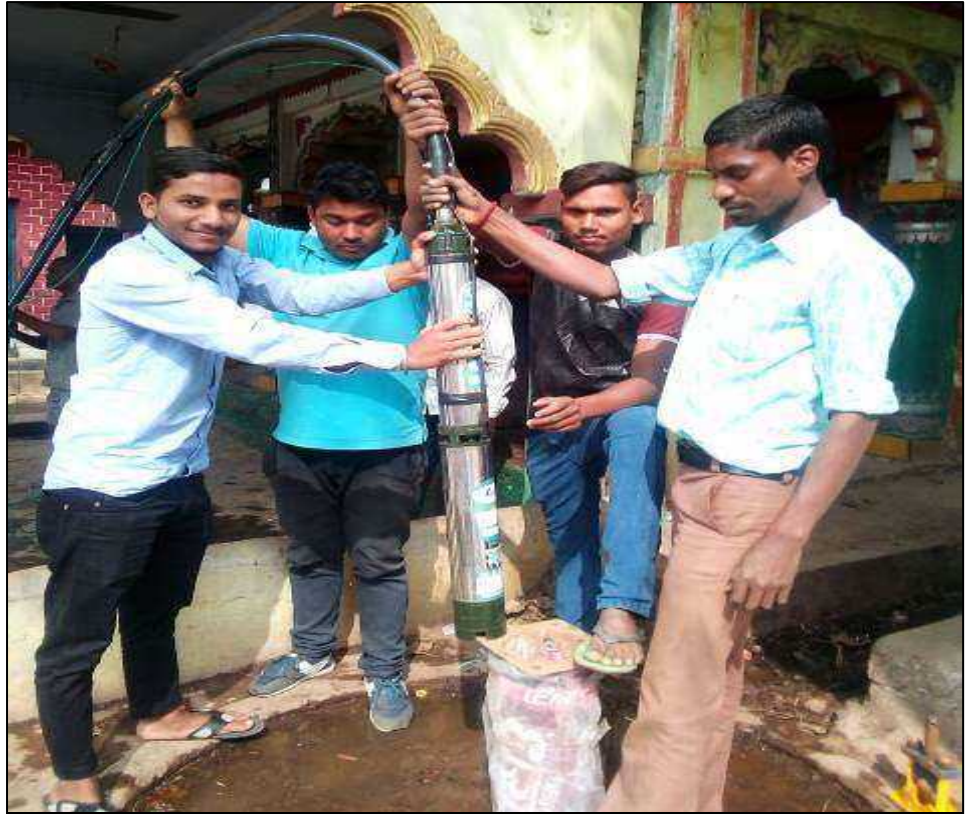
Submersible Pump (1 HP) Installation, Ward 12 Ram Gudi at Nariyara village
